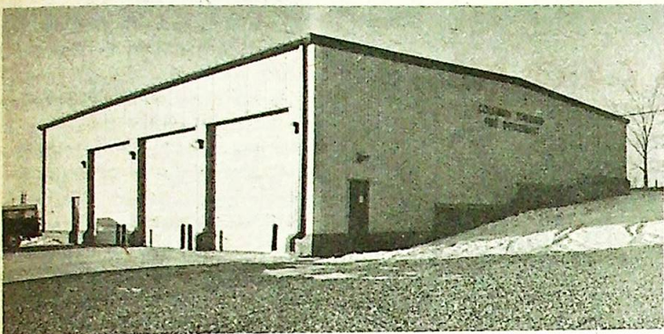
Columbia Township Fire Department's new 70' by 72' station. Built at a cost of $250,000, it has 3 double bays, office space, restrooms, kitchen, and room for living quarters if ever needed.
