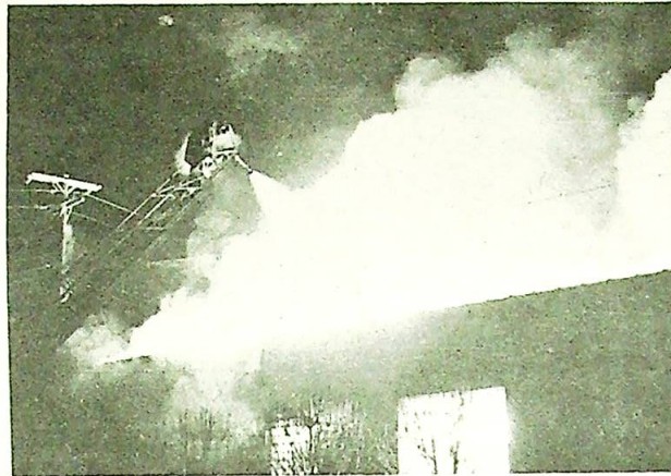
An early morning blaze at the Elks Club destroyed all but the front most portion of the building and kept Rushville City firemen and 10 volunteer fire departments on the scene for almost an entire day. The fire originated in the east corner of the kitchen area in the basement. Units from Rushville Twp., Raleigh, Glenwood, Milroy, Arlington, Carthage, Morristown, Manilla, Jackson Twp. and the snorkel from Connersville F.D. fought the stubborn fire.
