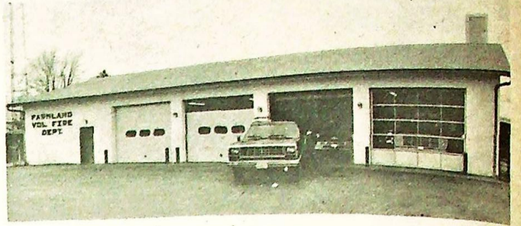
The Farmland Fire Department installed all new overhead doors to cut heat cost as well as dress up the look of the building. They suggest that if you have an all glass door that you look into this type of door. You won't believe the savings on heat bills next winter.
