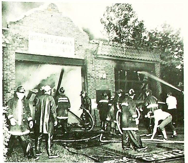
Remains of Beverly Shores Fire Station
