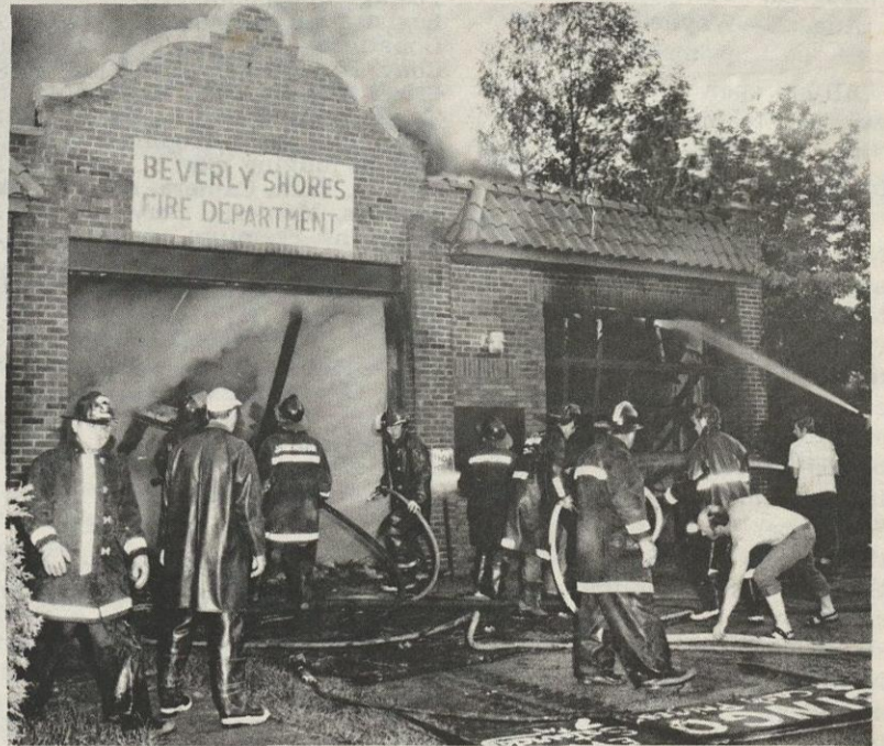
Remains of Beverly Shores Fire Station
