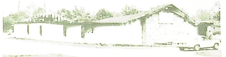
During a recent storm, this church in Wayne Township, Marion County was hit by lightning with these damaging results. Services were being held at the time but all escaped from the building.
