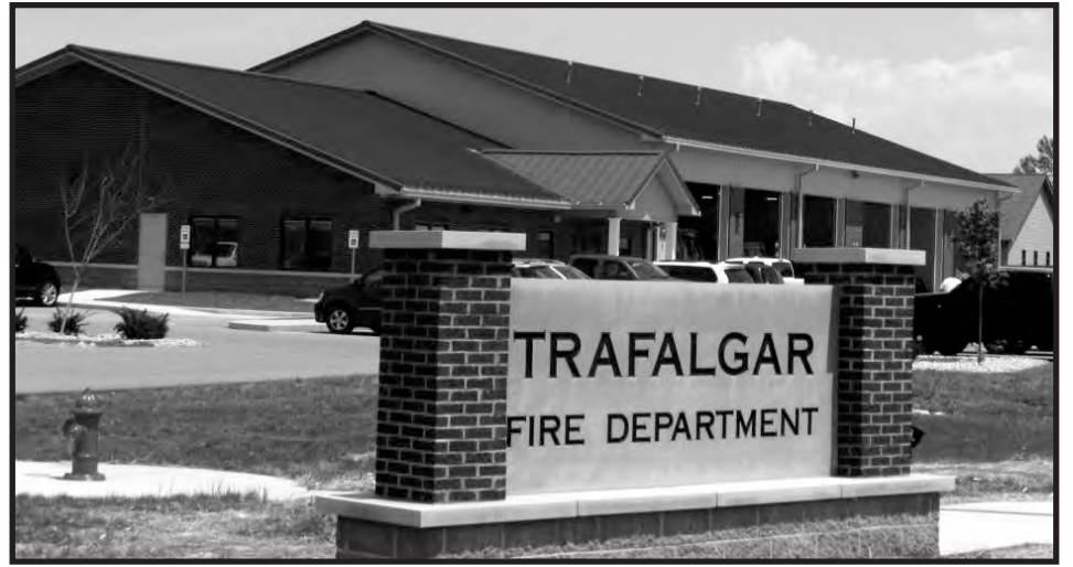
Newly constructed station of the Trafalgar Volunteer Fire Dept. in District 10.
