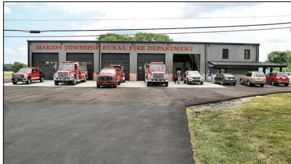
New Fire Station, Stoll Steel in Odon, IN was the general contractor. Open House Photos submitted by Peter Horton
