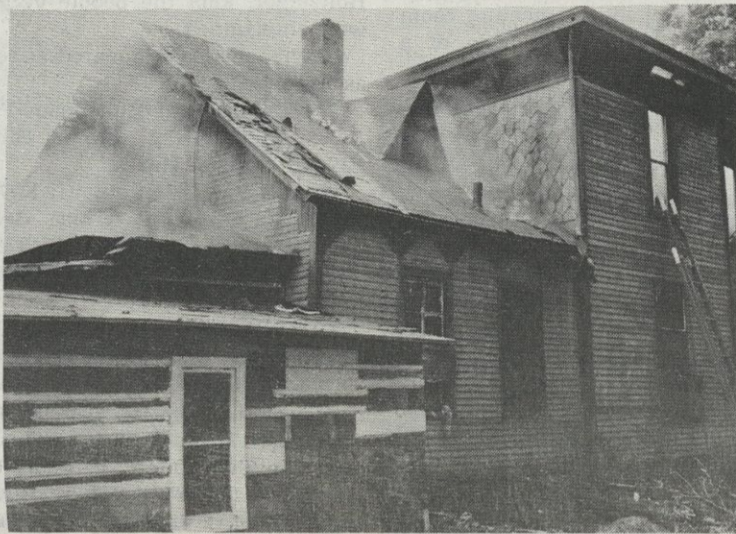
House badly damaged. Roof gone. Notice the fancy bric-a-brac and cornice.
