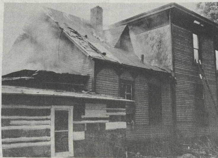
House badly damaged. Roof gone. Notice the fancy brick-a-brac and cornice.
