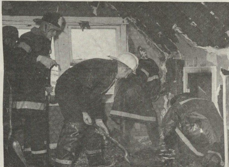
Firemen from Pike Township perform salvage and overhaul after confining fire to one room.
