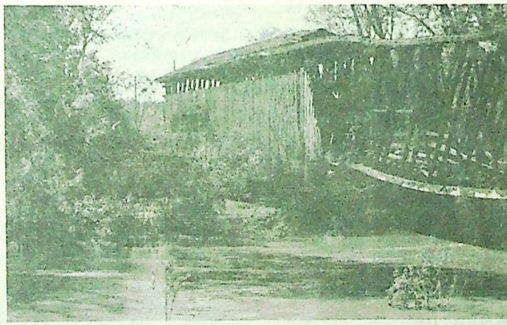
South end of Bridge looking South
