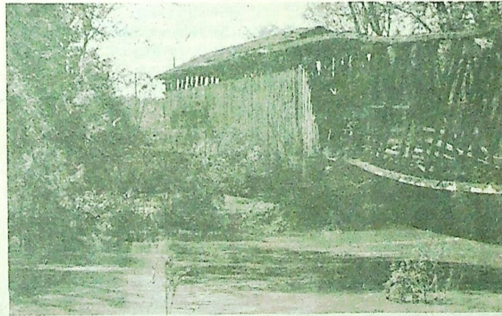
South end of Bridge looking South
