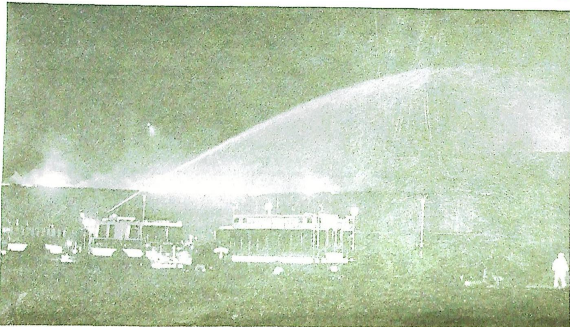
Southern Wells Elementary School Fire Scene
