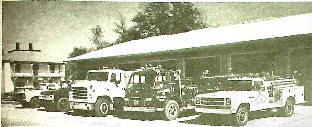
Equipment of Paragon Fire Dept. in front of new station.
