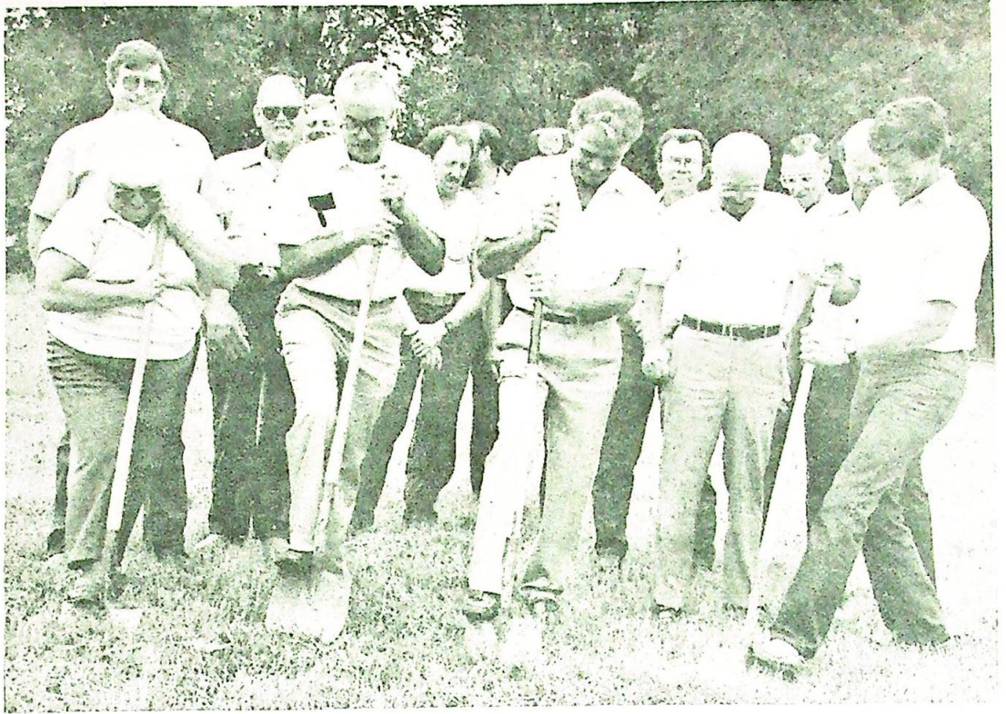
Hancock County - The Green Township fire department recently broke ground on a 4-bay, 40 x 80 building located at State Roads 9 and 234. The picture includes the trustee, contractor, I.M.I. owners, advisor board members and firemen.
