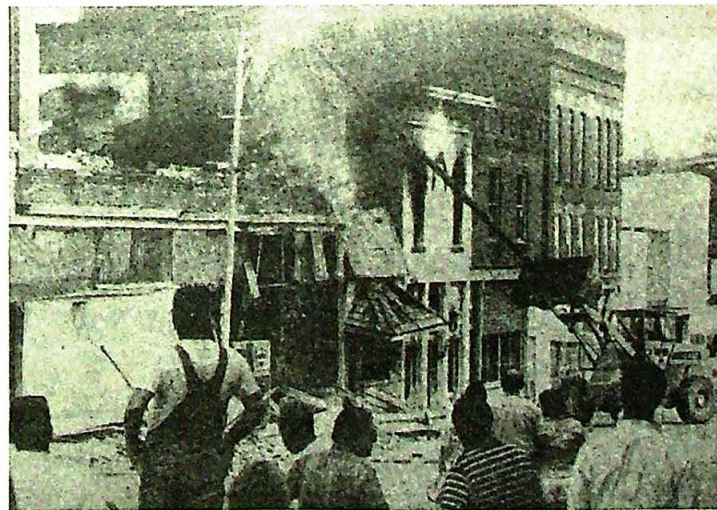
Nearly 300 residents of Williamsport turned out Wednesday afternoon to watch as Jimmy Taylor of Attica knocked down some burned-out downtown buildings. A fire Monday morning destroyed the town's only hardware store, a beauty shop, a barber shop, the offices of two lawyers and the offices of the Warren County school corporation, all in a block of North Monroe Street.
