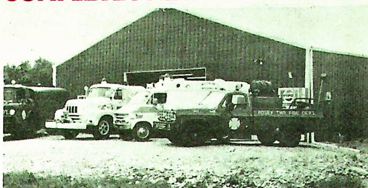
View of the new 30 by 40 structure erected by the volunteer firemen to house the Posey Township Volunteer Fire Department
