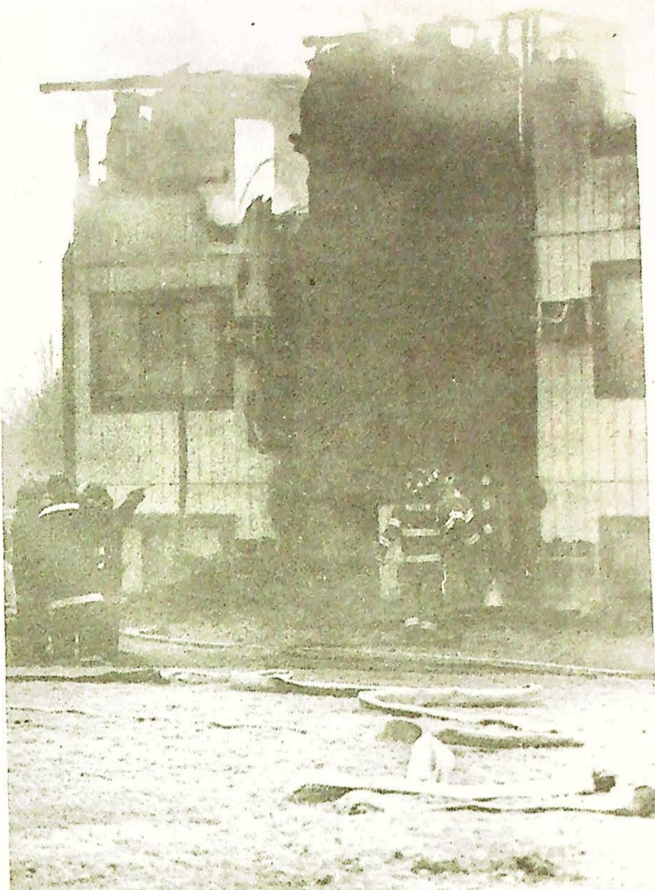
Firefighters survey damage after Michigan City apartment fire guts building.
