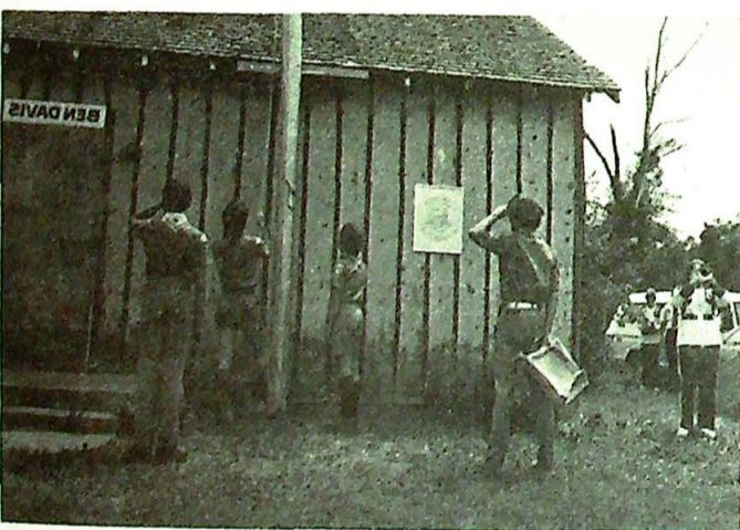
Taps for the old Ben Davis Train Station before demolition for souvenir sales
