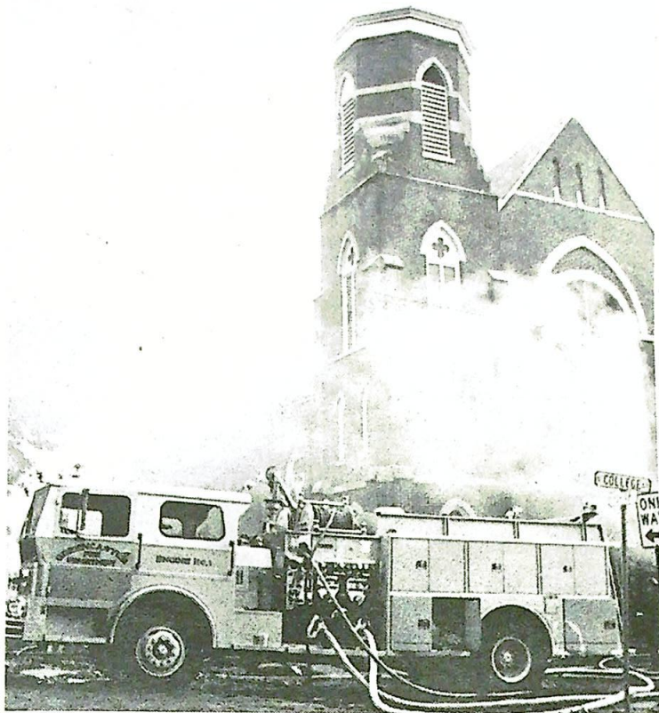
Struck by Lightning, Church is a Total Loss
