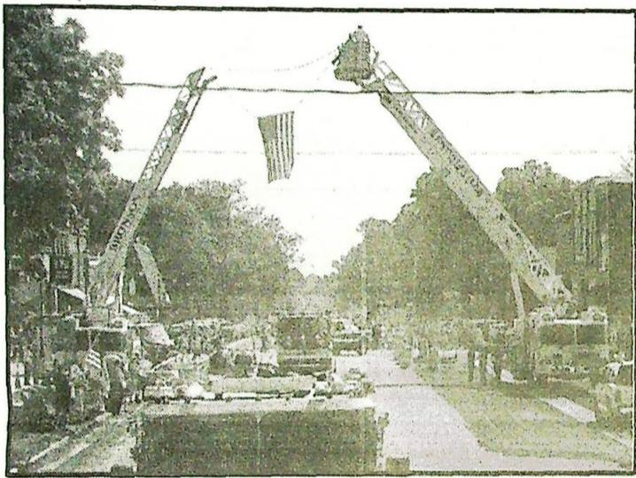
Transporting the Twin Tower Beam to Osolo Township Fire Department.
