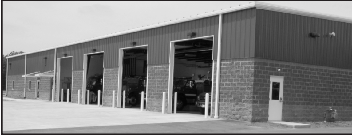
Pictured above – District 10 Morristown Volunteer Fire Department's new station just off Highway 52 in Morristown, IN.
