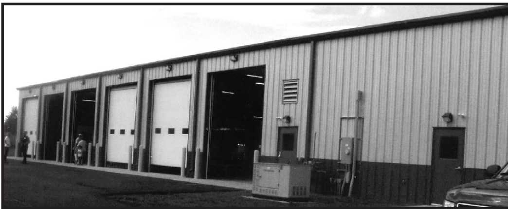
New fire station
