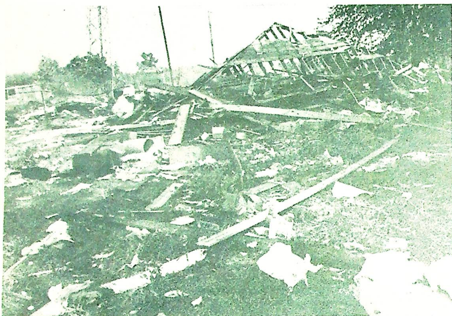
Damage was extensive in the July 28th fatal explosion of propane gas.
