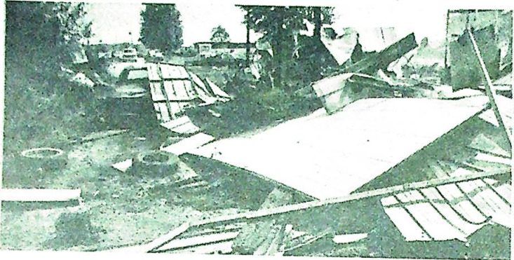
Destruction from the Bloomington explosion. See page 1.
