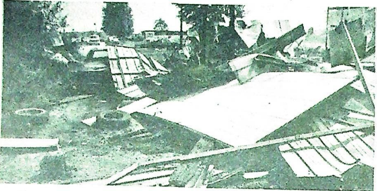
Destruction from the Bloomington explosion. See page 1.
